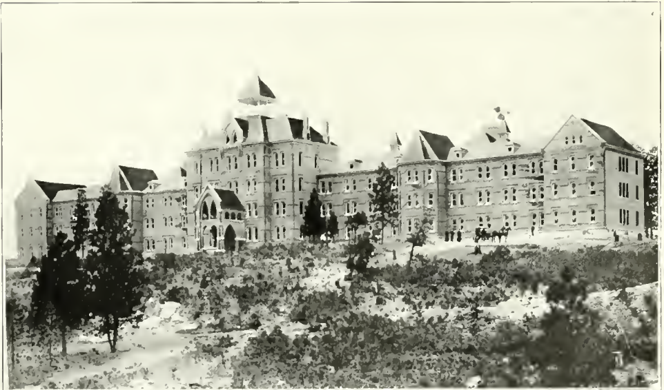
STATE HOSPITAL FOR THE INSANE AT MEDICAL LAKE
